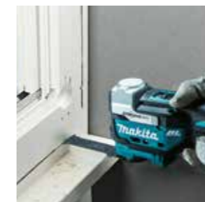
Removal of window frame
