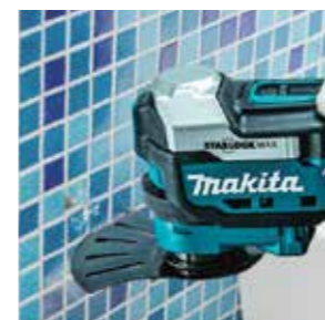
Routing joints on wall tiles
