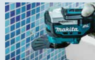
Routing joints on wall tiles
