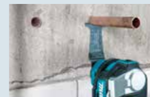
Copper pipe flush cutting
