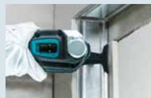
Door opening work
