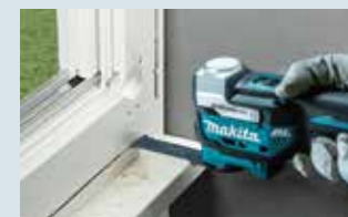
Removal of window frame
