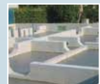
Small work area
