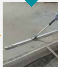
Leveling with the screed
