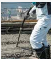
Compacting with a vibrator
