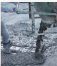
Unloading fresh concrete
