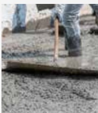
Spreading the concrete
