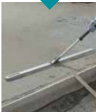
Leveling with the screed
