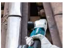
For railway maintenance work
