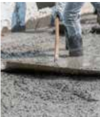
Spreading the concrete
