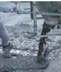
Unloading fresh concrete
