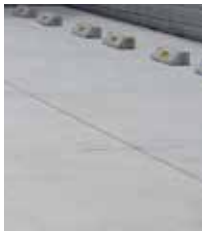
Completed after curing
