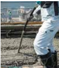
Compacting with a vibrator
