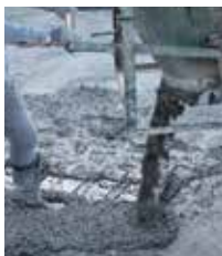
Unloading fresh concrete
