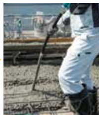
Compacting with a vibrator
