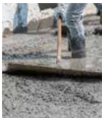
Spreading the concrete
